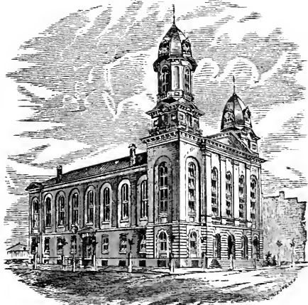
CLINTON COUNTY COURT HOUSE, LOCK HAVEN.
